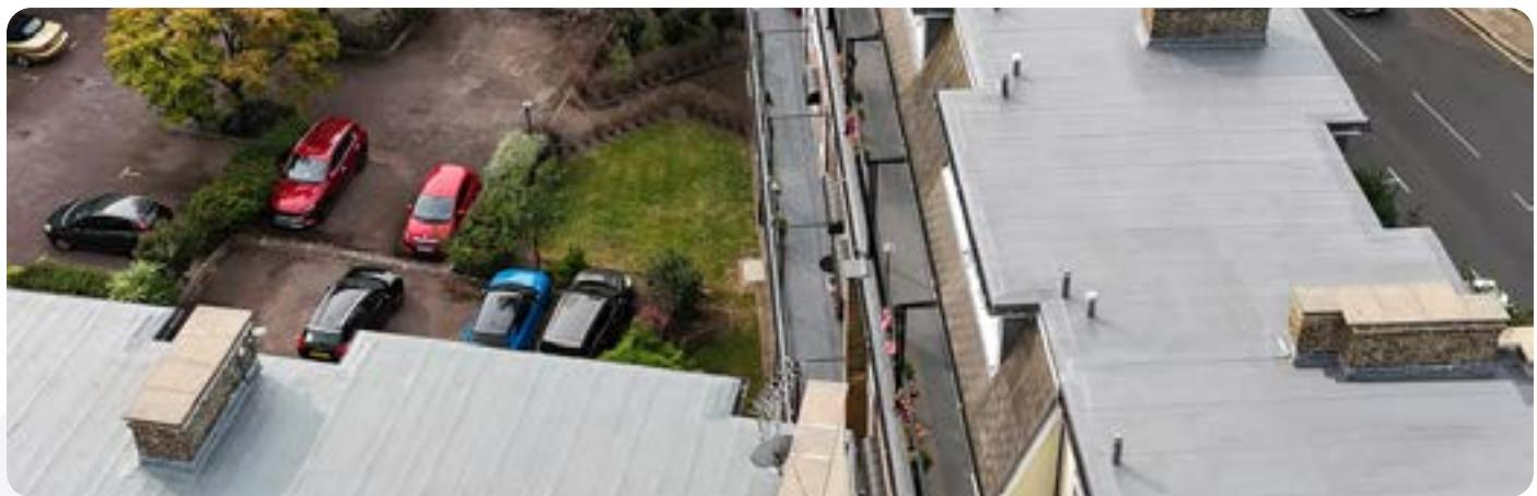
For balconies and communal walkways, Garland UK specified the Dura-Walk system. Approximately 1,500 m<sup>2</sup> of walkways and balconies were refurbished. Adhesion testing was carried out prior to installation due to previous low-level liquid applications showing early signs of failure. The new Dura-Walk system delivered a durable, anti-slip finish suitable for both private balconies and high-traffic communal areas.
