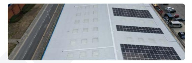
Adding to the challenge, the project needed careful coordination to ensure minimal disruption to tenants. For example, the inverters were designed to be mounted externally in a protective cage. The works had to resolve leaks, manage asbestos risks, improve thermal performance, and support the solar array, all without disrupting tenants.
