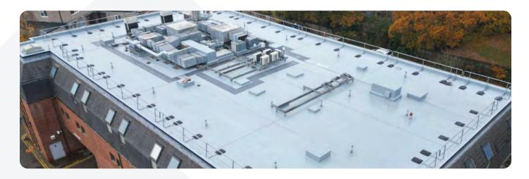
Located in Enfield, **The Cavell Hospital** is a key facility for **Circle Health Group**. Spanning over **1,000 square metres**, the building's existing mastic asphalt roof had reached a critical state of disrepair, causing water ingress and internal damage.
