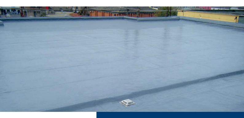
Liqui-Zero is a two-component liquid waterproofing membrane specifically designed for application in sensitive environments.
