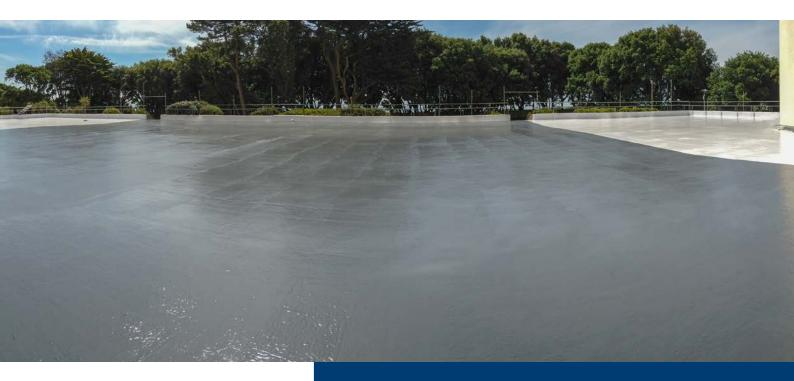
White-Knight is a multi-purpose single component polyurethane liquid-waterproofing membrane that can be used to coat the entire roof or restore and repair single-ply, metal, asbestos or modified roof systems.
