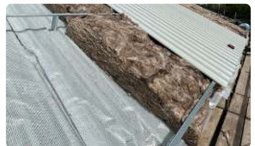
Twin skin R-MER CLAD installation allowing for insulation within the void.
