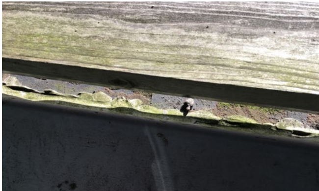
Peeling flashing
