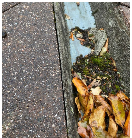
Poor drainage and blocked gutters
