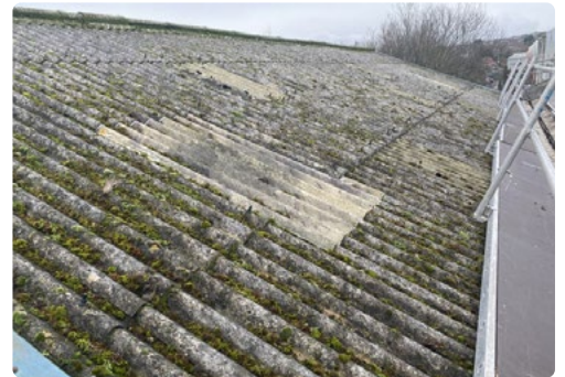
Preparing asbestos roof for encapsulation
