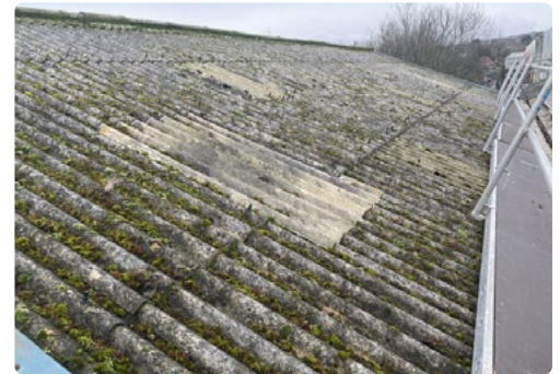
Preparing asbestos roof for encapsulation
