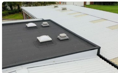
Final R-MER CLAD and StressPly Flex installation
