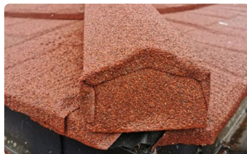
Final R-MER TILE ST installation
