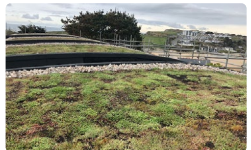
Final StressPly Flex Plus installation
