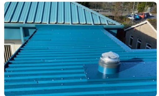
Final StressPly Flex and R-MER CLAD installation
