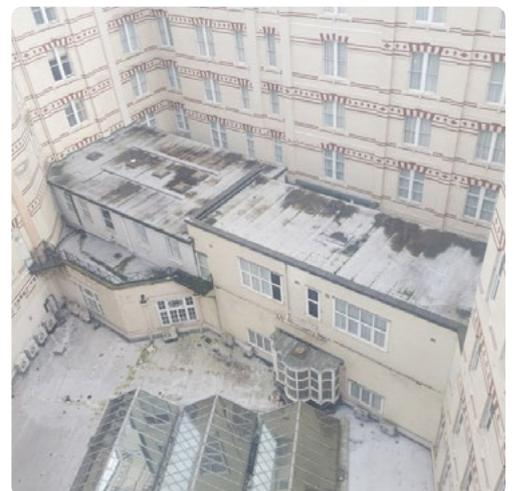
*The original single-ply system had failed across the courtyard and atrium roofs, leading to the insulation becoming fully saturated with water.*
