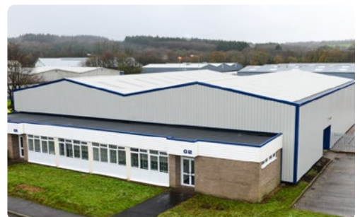
Final R-MER CLAD and StressPly Flex installation
