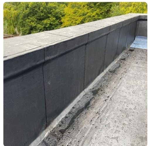
After thoughtful consideration, an inverted roof was selected for high-performance waterproofing, whilst allowing for easy access and maintenance by the facilities management team.
